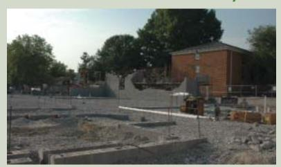
Blocks outline hallways and rooms of the first level as workmen start on the first exterior walls of the building. Hughes Hall is visible behind.
