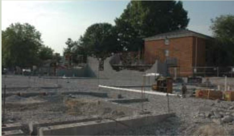
Blocks outline hallways and rooms of the first level as workmen start on the first exterior walls of the building. Hughes Hall is visible behind.
